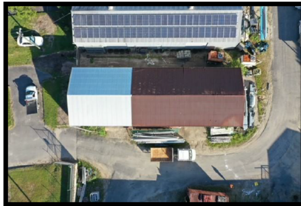
Work Shed Roof reconstruction
