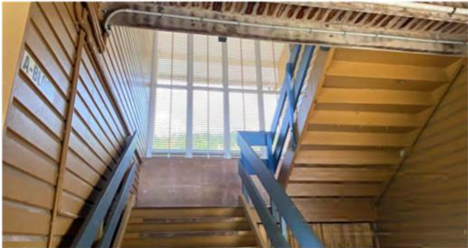
Staircase G block
